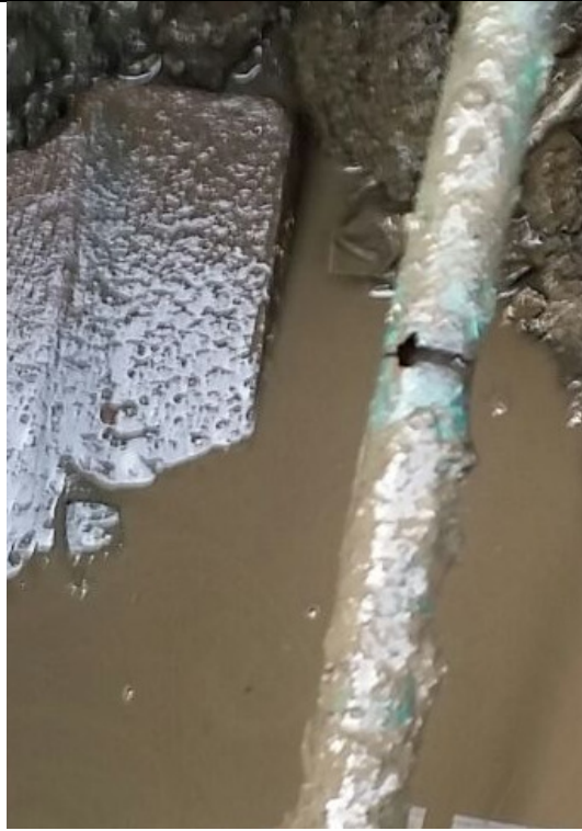
Maynooth - Pin-hole Leak (1.4m 3 )
