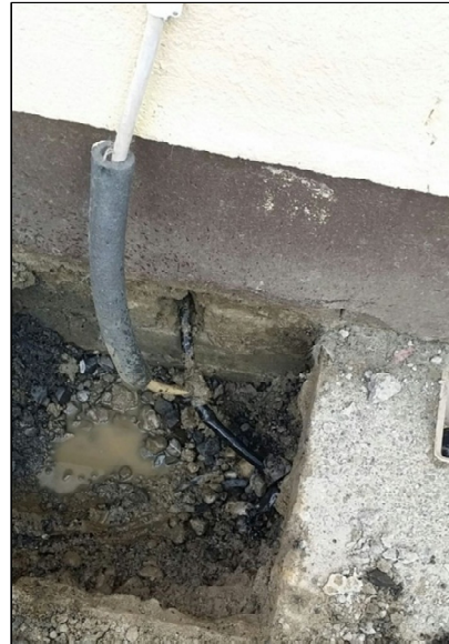
Leak - Poor Quality Plumbing
