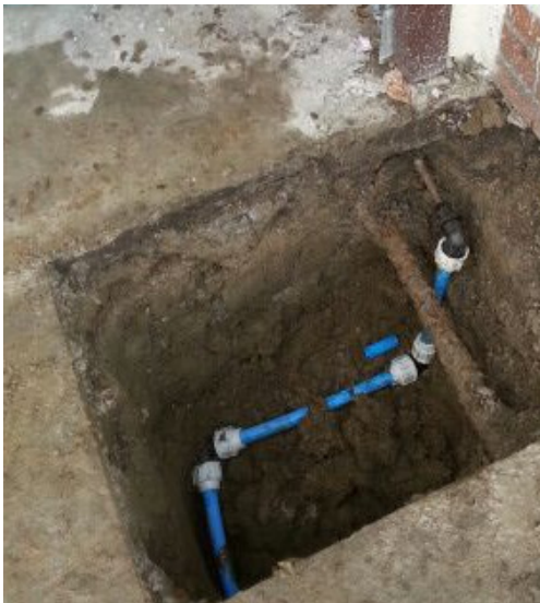
Leak at point of entry
