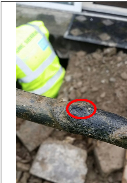
Maynooth - Pin-hole Leak (1.4m 3 )
