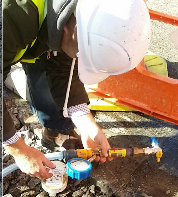
Pressure Test – Post Repair
