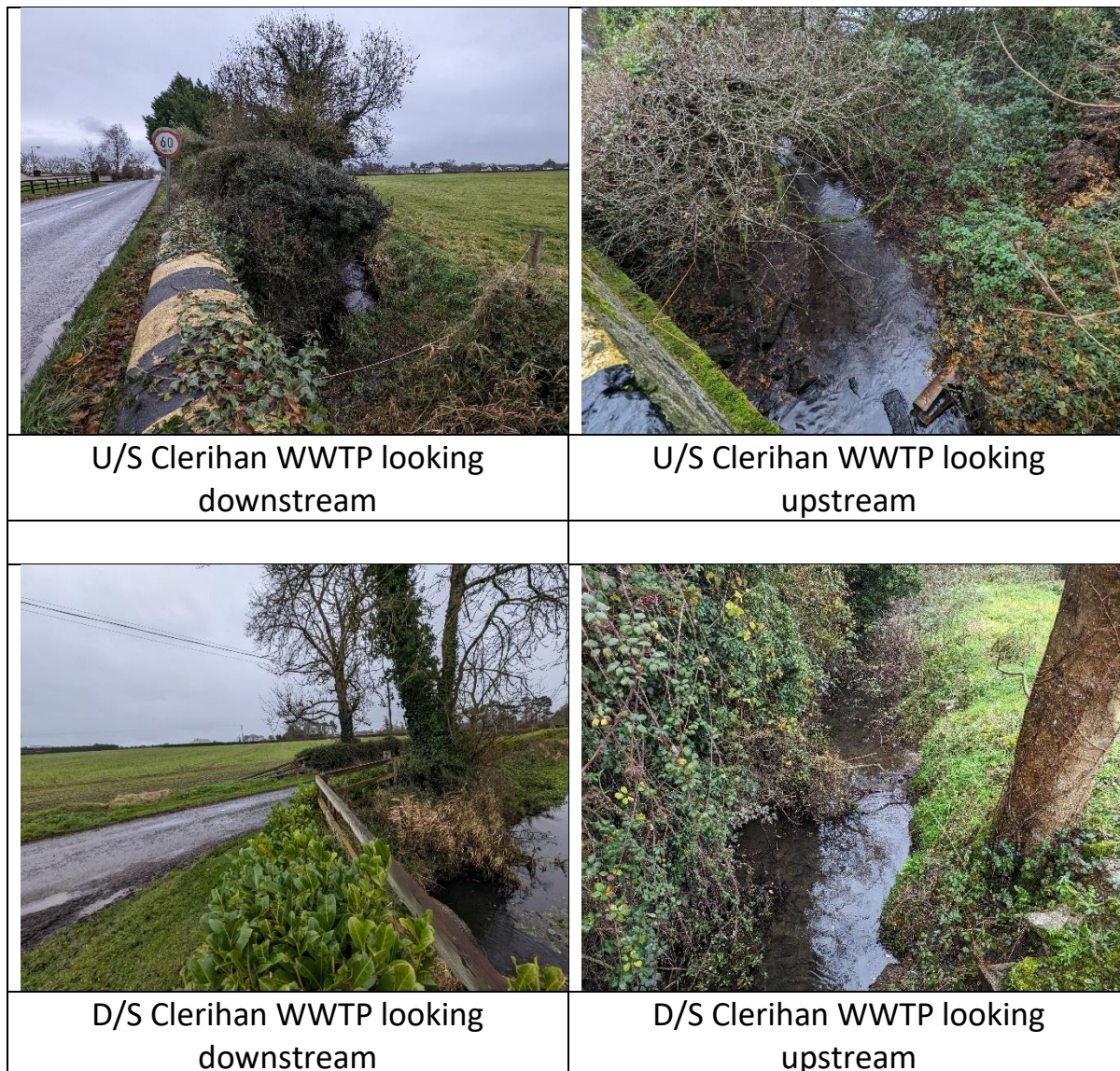
Figure 2. Upstream (U/S) and downstream (D/S) of Clerihan WWTP.
