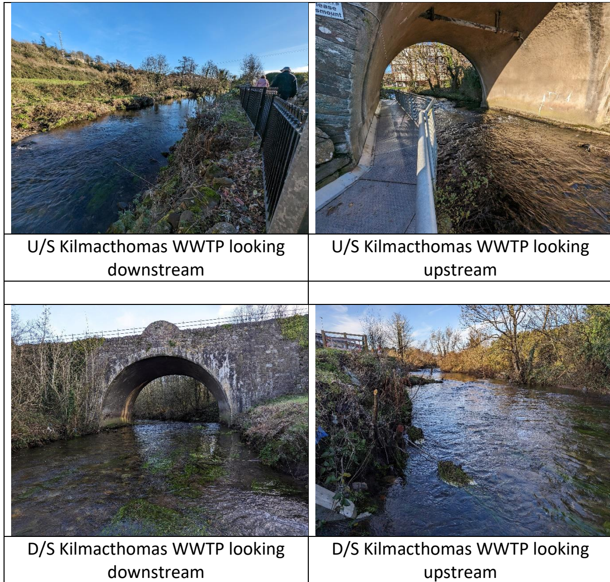
Figure 2. Upstream (U/S) and downstream (D/S) of Kilmacthomas WWTP.
