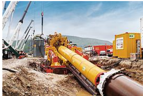
Figure 26 Herrenknecht Direct Pipe® system
