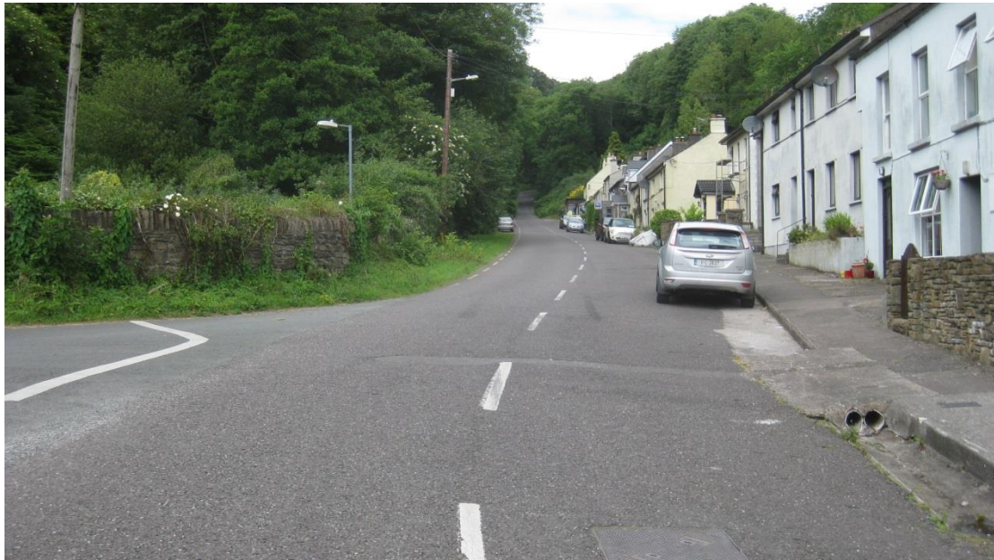
Figure 7 - Glen Road looking northwest
