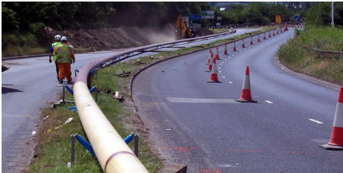
Figure 6 - Pipe laydown example (Image A E Yates)
