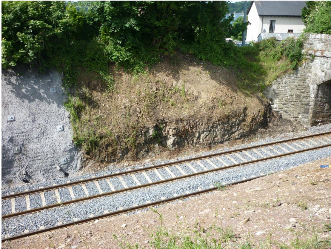
Photo A7/2. View westward of the railway section on the eastern side of Bridge 2. The bedding dip is towards the left (i.e. to the south-southeast).
