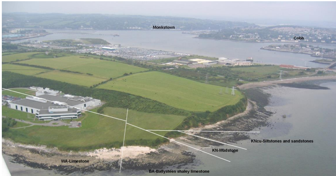
Appendix B2. Aerial view of the Ringaskiddy coastal section showing the bedrock.
