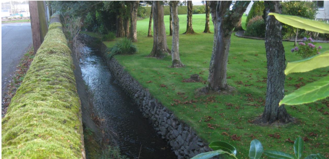
Figure 9 - Water course and low lying gardens adjacent to Glen Road
