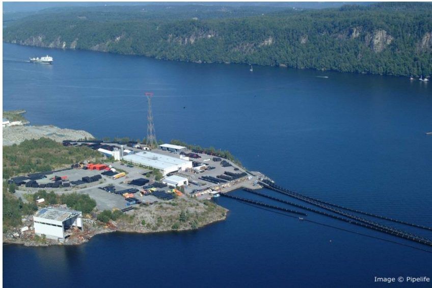
Figure 11 - Pipelife extrusion facility, Norway
