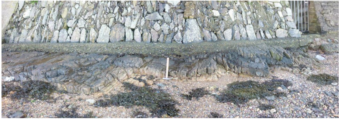
Photo A6/4. Bedrock 5. 50-60m Undulating beds in sandstones of the Cuskinny Member. The beds are extensively fractured by a vertical fracture cleavage and intense jointing.
