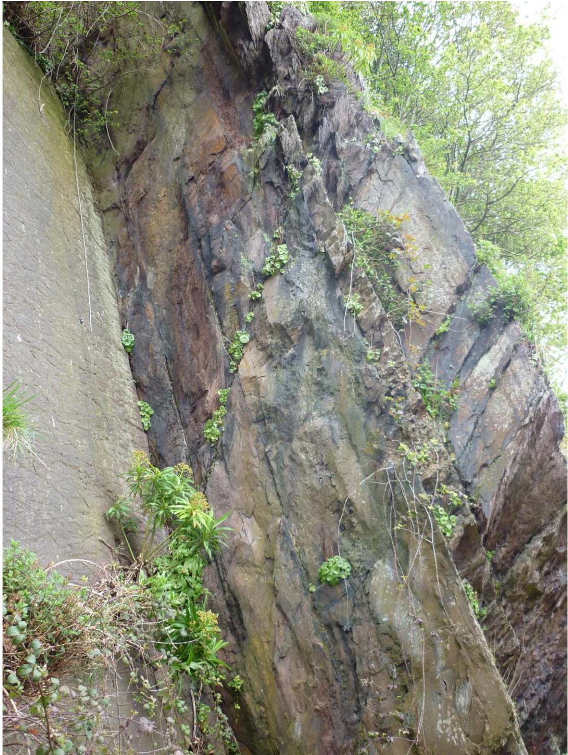
Fig 13.10. Gyleen Formation at Glen Road Quarry (lower). The surface in the centre is a joint plane. The pale coloured surface on the left side is a bedding plane. Facies 2- Well-bedded alternating purple sandstones and mudstones. Bedding planes dip steeply to the right (southwards).
