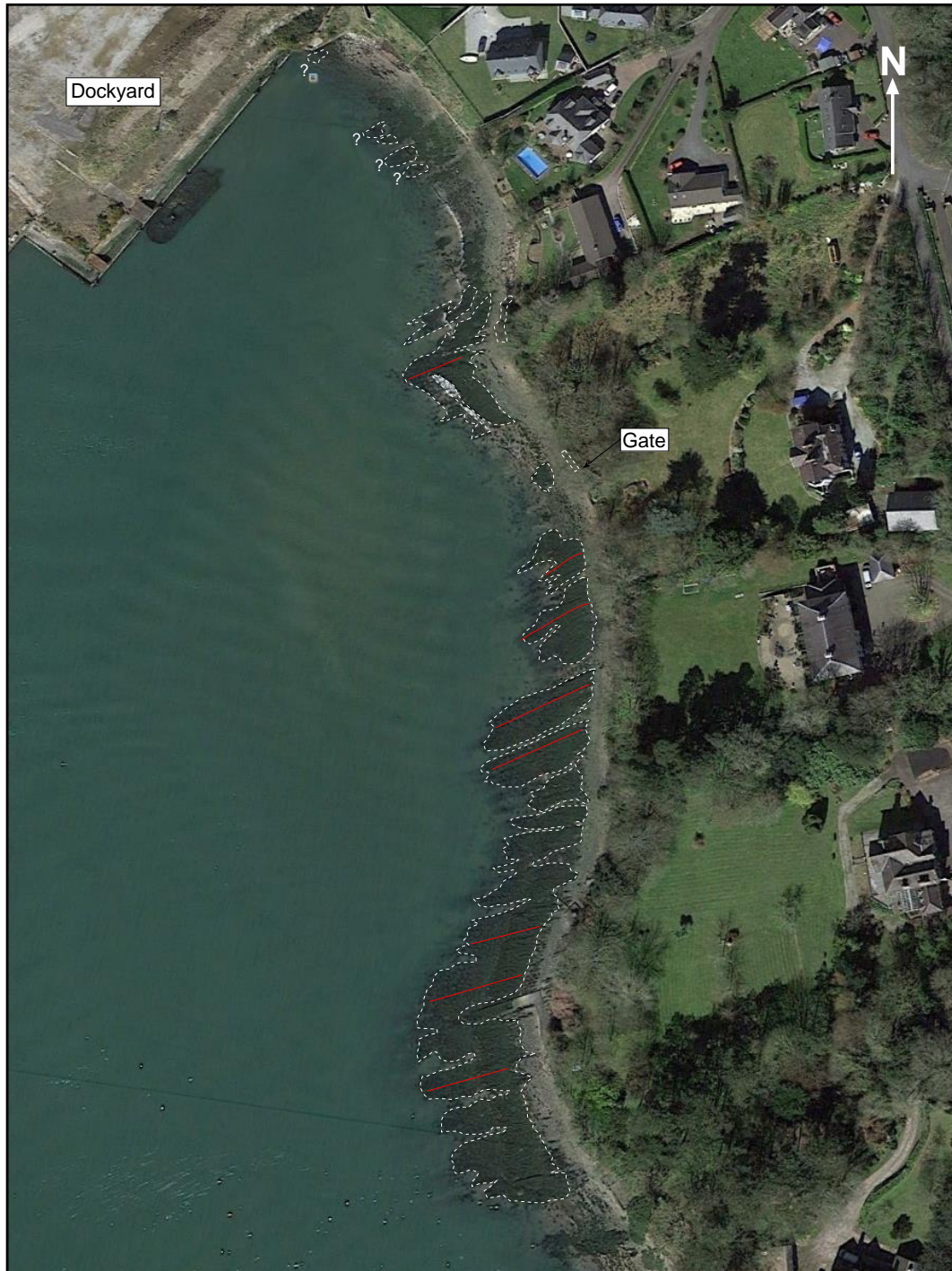
Photo A6/1a. Aerial view of Ringacoltig coastal zone showing approximate areas of bedrock outcrop outlined in white line. Strike of bedding/cleavage shown in red. Image Google Earth .
