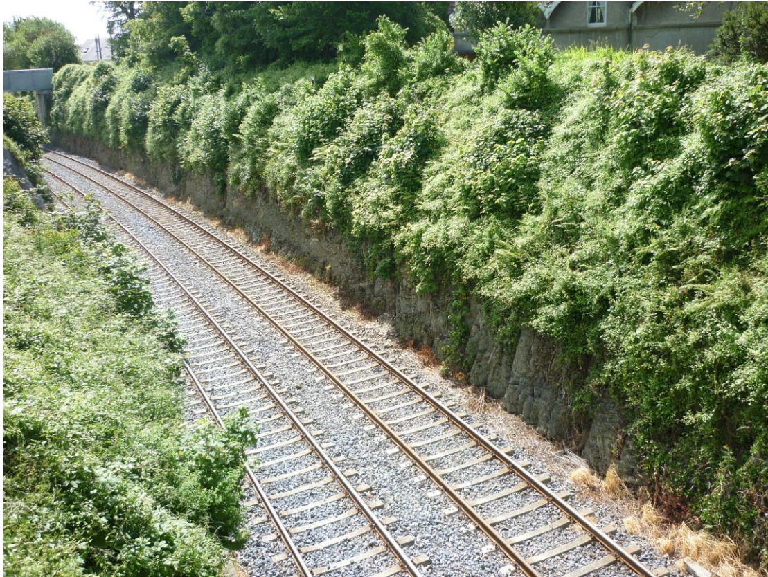
Photo A7/3. General view south-southeastwards taken from Bridge 3 towards Bridge 4 showing the outcrop of the Cuskinny Member which shows extensive closely-spaced jointing here.
