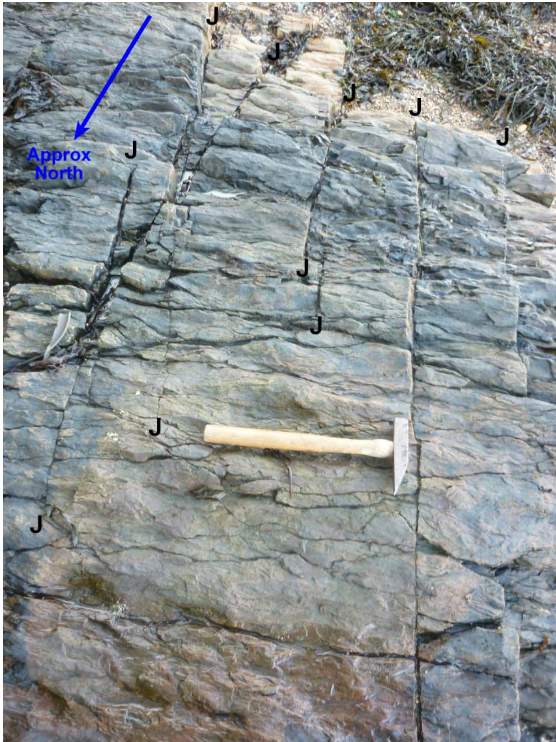
Photo A6/7. Intersecting joint sets in fractured sandstones of the Cuskinny Member at Ringacoltic shore north. The fractures parallel to the hammer shaft are a fracture cleavage. This is a widely spaced cleavage that persists through sandstones. Note that some of the joints are laterally discontinuous. The top surface of the bedrock here is a bedding plane.
