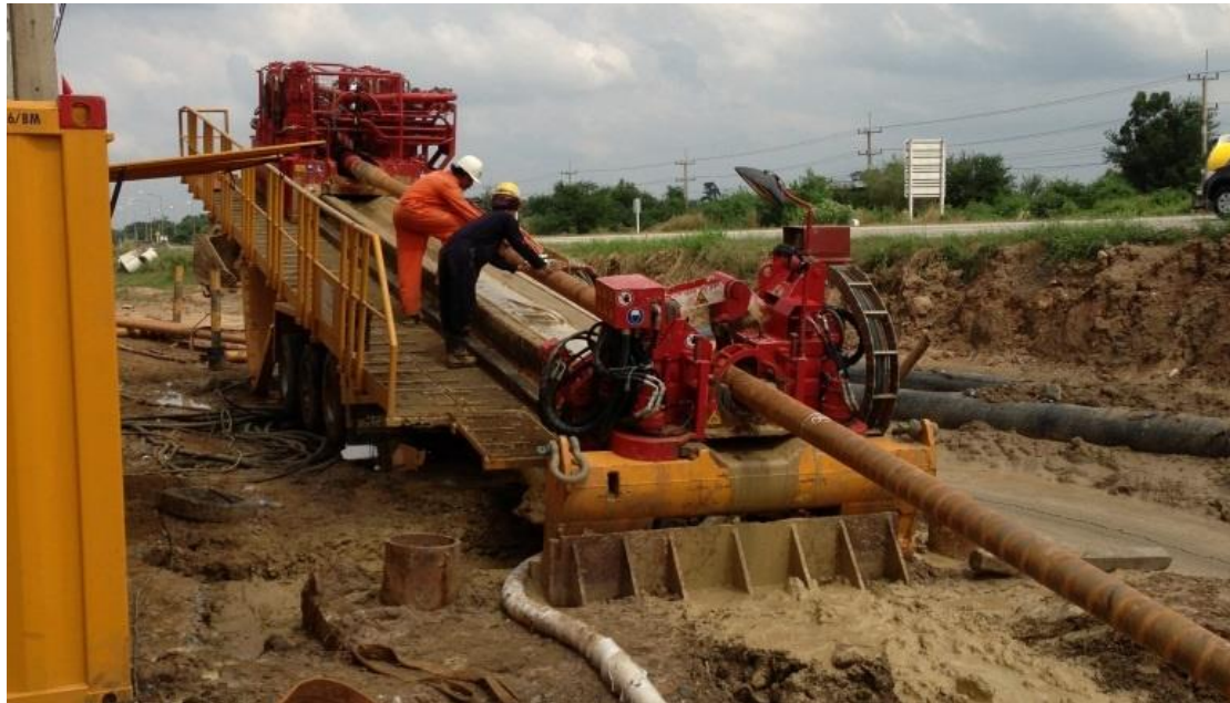
Figure 20 - Horizontal Directional Drilling Rig (Thailand)
