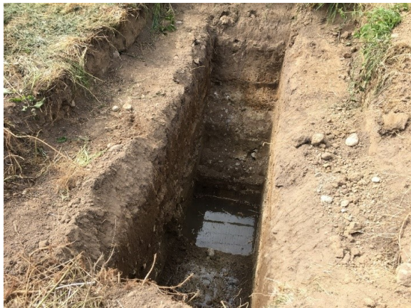
Example of a trial pit survey.
