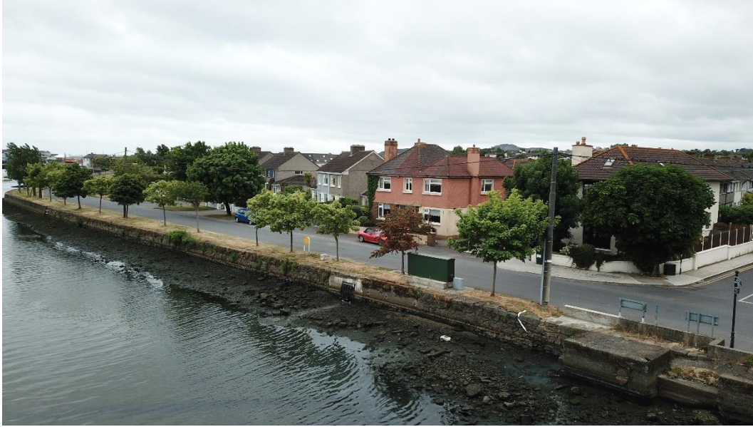
Figure 2.5: South Quay (viewed from the river channel)
