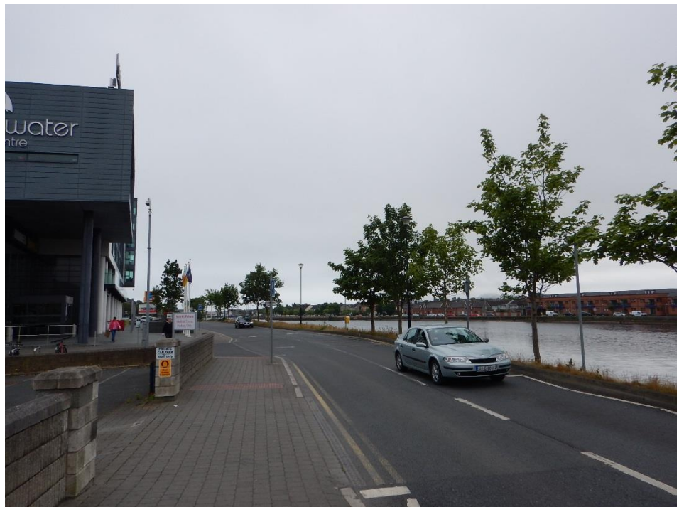
Photo 4. Young trees established in the verge along the northern bank of the river, south-east of the road bridge
