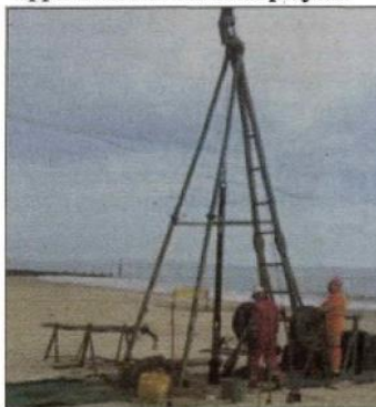
Marine investigations at Portmarnock.
