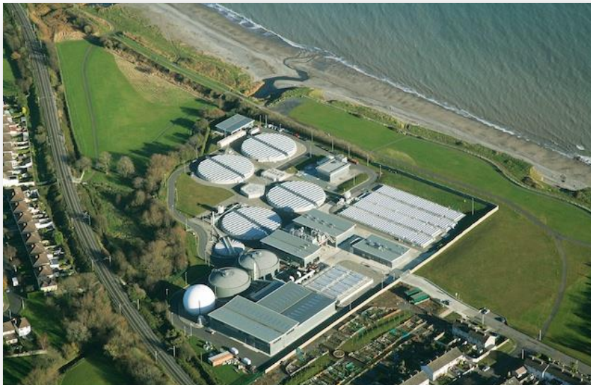
Figure 2-5 Shanganagh-Bray Wastewater Treatment Plant, Shankill
