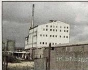
The plant will be built on the site of the old Wallboard site.
