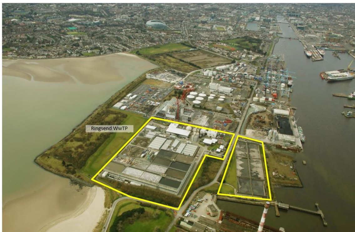
Figure 1-1 - Ringsend Wastewater Treatment Plant
